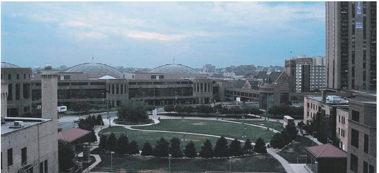
Previously, the Minneapolis Convention Center had to turn down business, but thanks to its recent expansion, it can now host numerous events. (Photos courtesy of Carlisle Coatings & Waterproofing, Inc., Wylie, TX.)
